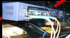
Extreme switch with 2 ten gigabit uplinks
