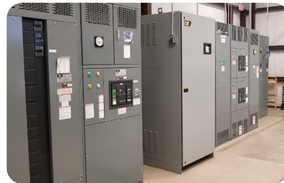
MCC Panel and Automatic Transfer Switch
