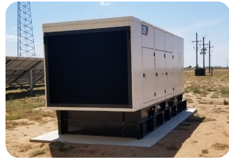
500kW Backup Diesel Generator
