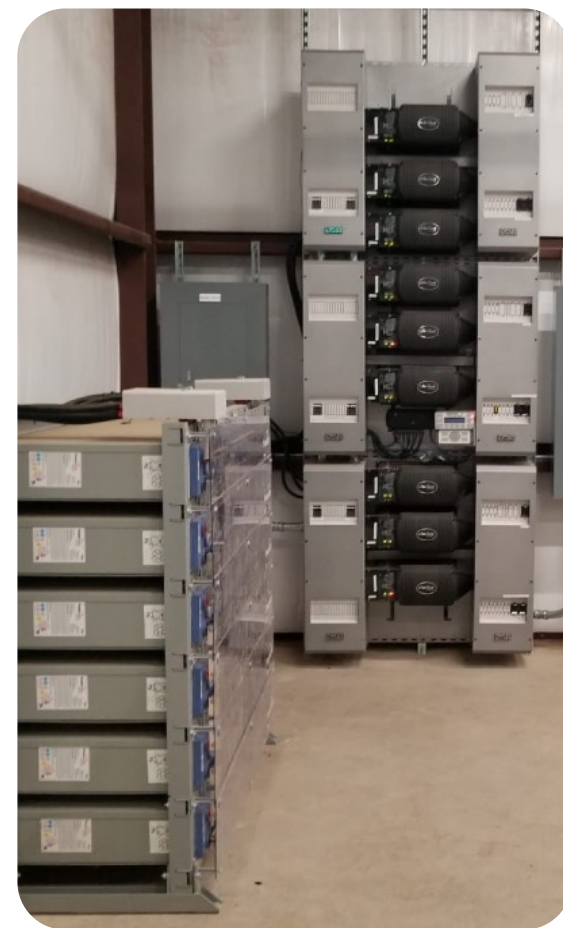
30kW Outback Inverters System with 48V / 1600Ah Lead Acid Battery
